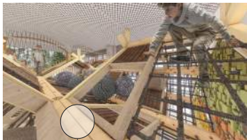
Steel structure, clad in wood
